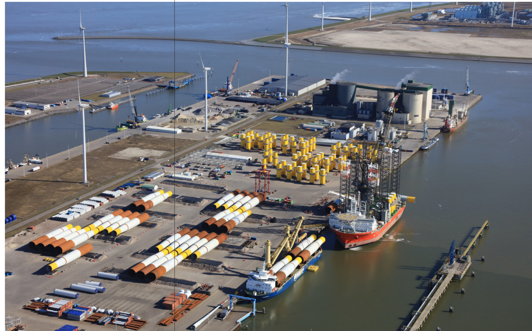
Offshore wind Eemshaven (photography: Groningen Seaports)
